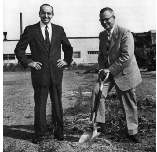
Figure 3. Sam Labate and Bob Newman breaking ground in 1959 for an addition to BBN's 50 Moulton Street building in Cambridge, Massachusetts. (Photo courtesy of BBN Technologies.)
